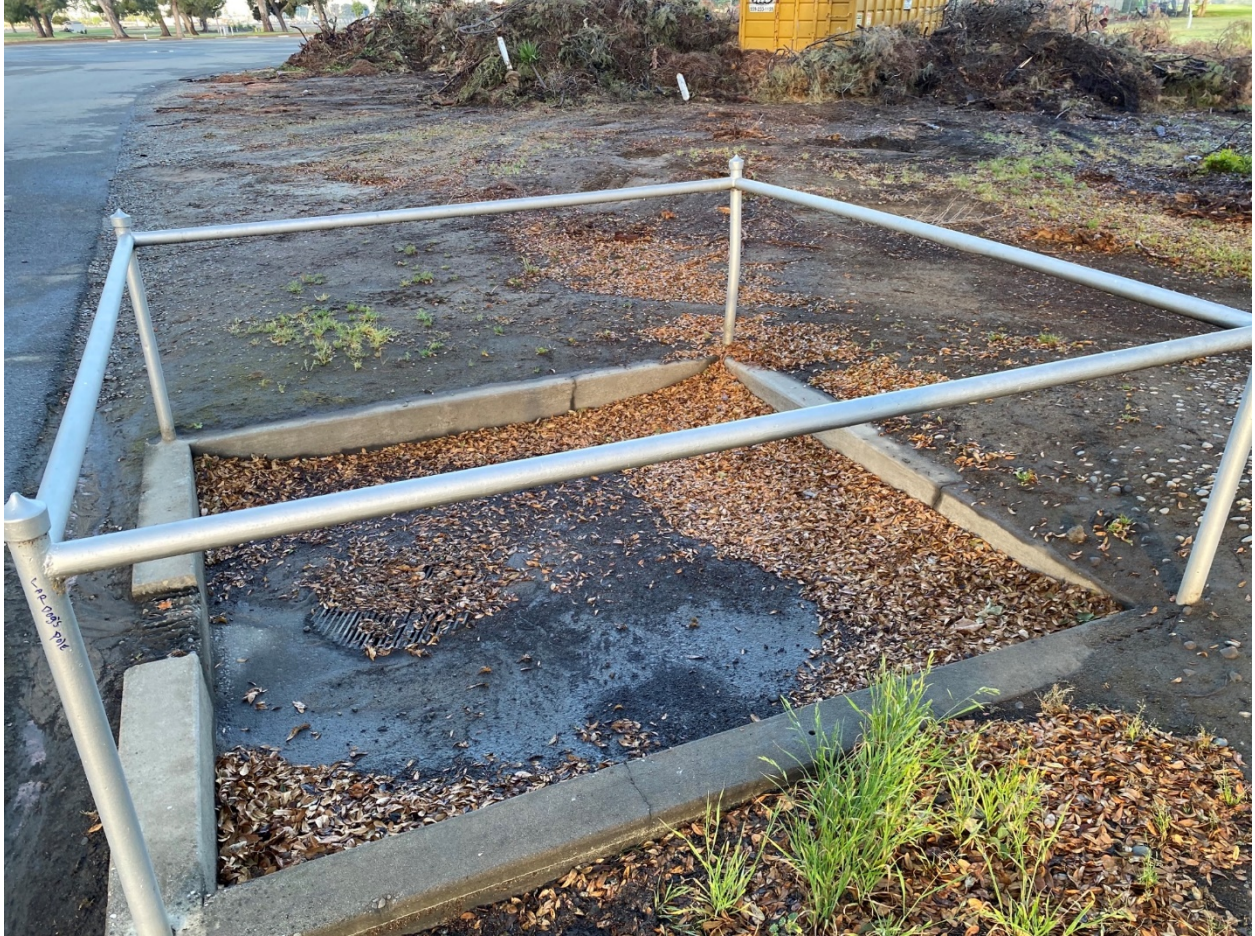
Photograph 11. Water Drainage Feature.
